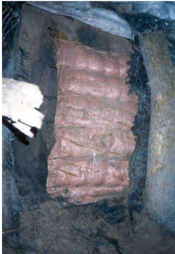
Figure 4. Note bulging of backfill between layers of reinforcement, indicating that the FILPAK is accepting the stress.
