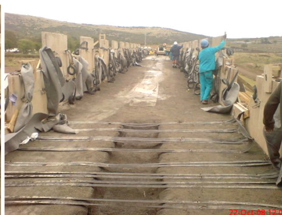
Figure 8 Gcuwa Dam: Excavated trench
