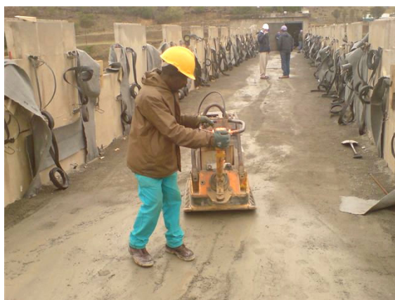
Figure 7 Gcuwa Dam: Compaction of MSE
